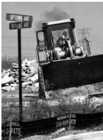
Uptown removes and rebuilds sidewalks to comply with the FHAA
